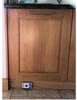
shut off if a leak is found, in locations where running interconnecting cables would be impossible or very difficult. The alarm unit will also provides both "Water On" and "Water Off" push buttons to allow the mains water supply to be turned off in an emergency of when the building is unoccupied such as going on holiday.
