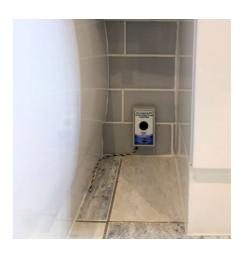
The RFWD8 has been designed to provide a water leak detection system with mains water supply
